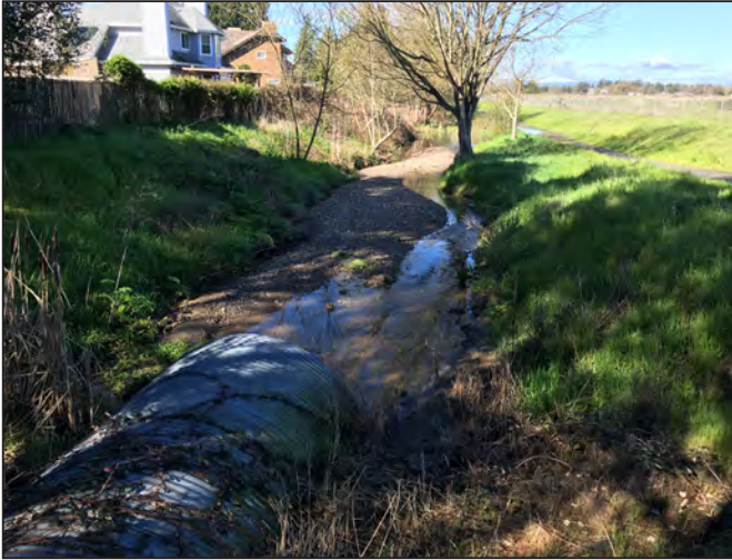
Photo a. Wilfred Creek at Snyder Lane crossing (March 2019) culvert severely blocked by chronic deposition, good site for targeted sediment removal.
