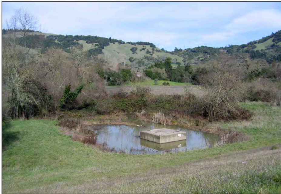
Photo a. Brush Creek Reservoir dam inlet structure with ponded water and some surrounding vegetation along creek above structure (Zone 1A).
