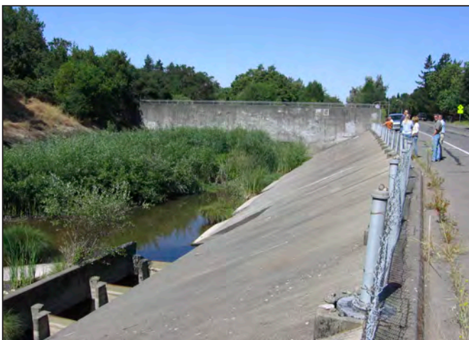
Photo e. Spring Lake Diversion (Zone 1A).
