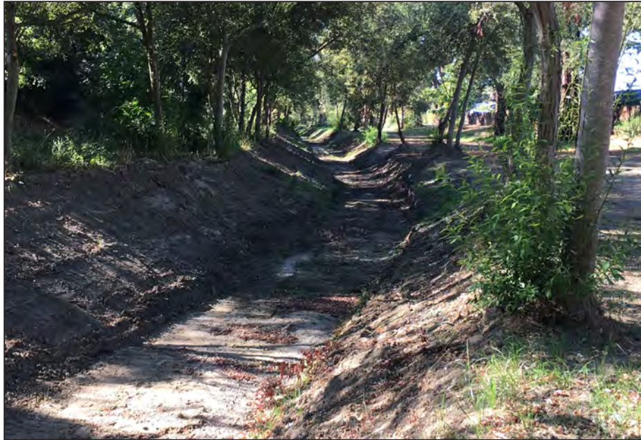
Photo a. Reach-scale sediment removal project at Five Creek (Reach 1) showing retention of mature riparian vegetation along the banks (October 2019)
