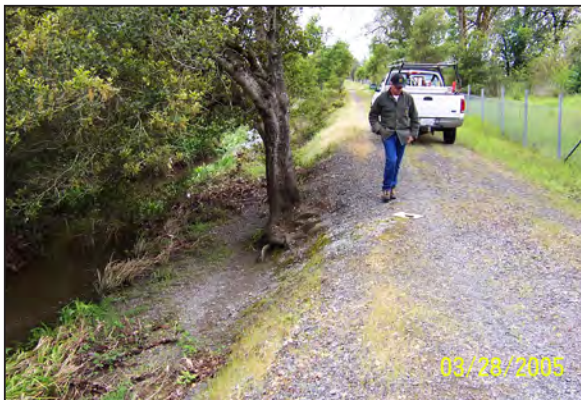
Photo a. Bank failure on Peterson Creek (Zone 1A).
