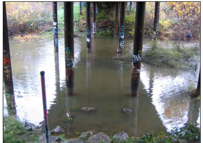
Photo d. Graffiti on bridge piling on Santa Rosa Creek at Willowside (Zone 1A).
