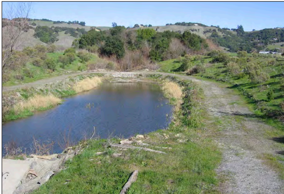
Photo b. Cook Creek Sediment Basin after being cleared of sediment.
