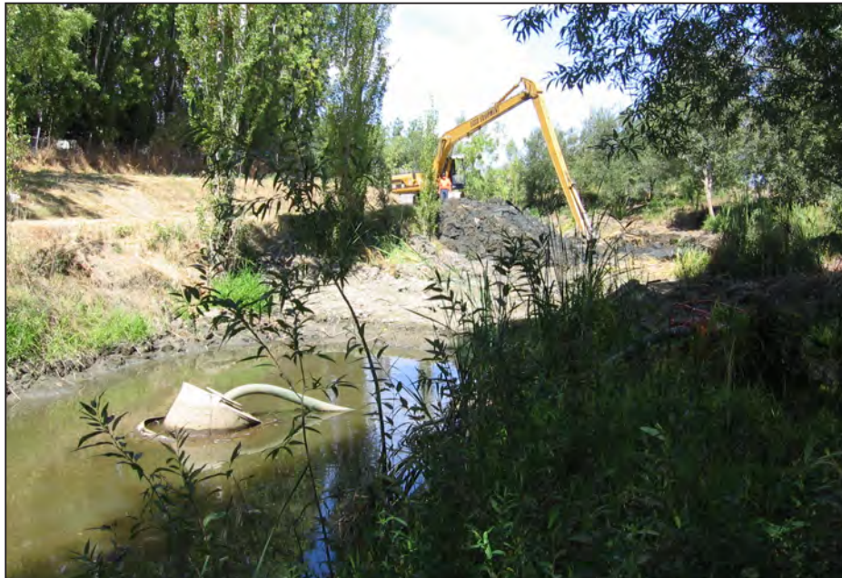
Photo a. Dewatering at Hinebaugh Creek sediment removal project (August 2008), intake screen and bypass hose seen in near ground, earthen berm damming flow seen just downstream of bypass hose, long-reach excavator shown in distance conducting sediment removal work from top-of-bank.
