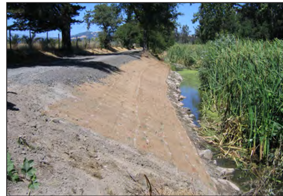
Photo b. Same site as Photo (a) after bank repair, prior to revegetation.
