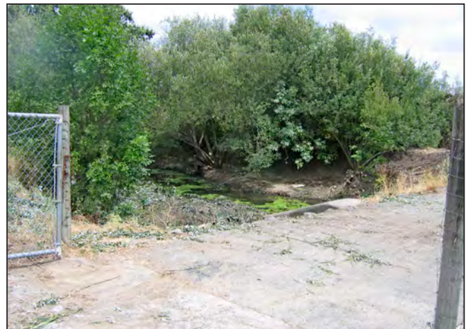
Photo f. Willows cleared from culvert outlet on Windsor Creek after maintenance (Zone 1A).
