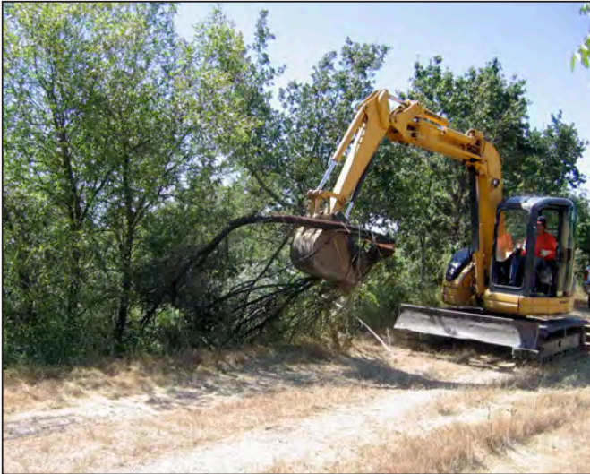
Photo a. Clearing cut brush with an excavator. Excavator is staged on adjacent access road.
