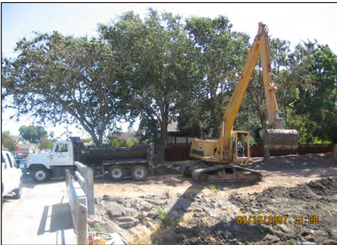
Photo c. Excavator positioned on access road on the top of the stream bank. Long-arm reaching into channel.
