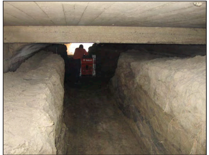
Photo b. Using a front loader to clear sediment in box culvert.
