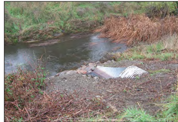
Photo b. Same site as Photos (a) after bank repair using minimum necessary rock rip-rap.
