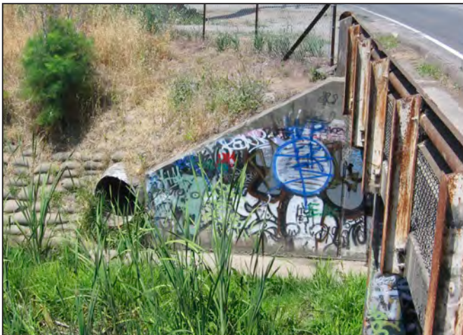
Photo c. Graffiti on bulkhead on Copeland Creek (Zone 1A).
