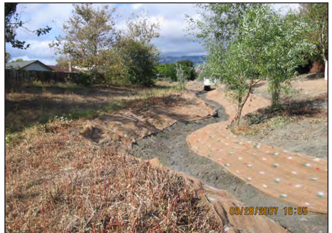
Photo f. East Washington Creek, looking upstream at Garfield Drive, after sediment removal project.
