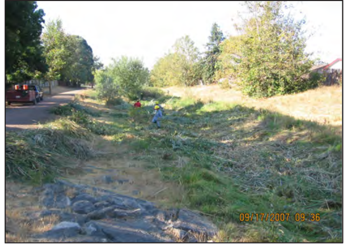
Photo b. Maintenance crew clearing vegetation by hand.
