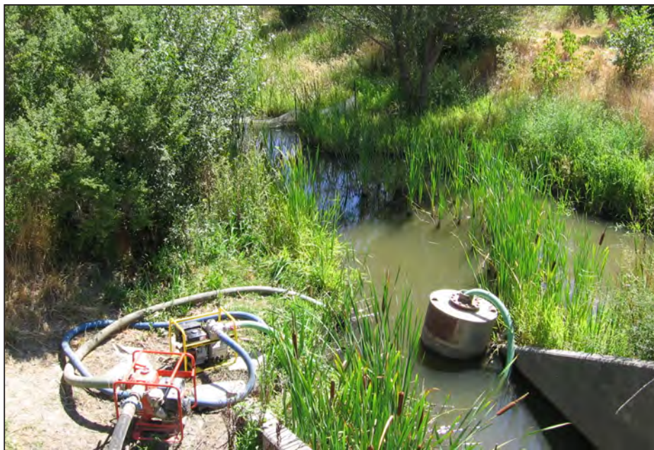
Photo b. Dewatering at Hinebaugh Creek sediment removal project (August 2008), upstream of dewatering reach shown in photo (a), intake screen, pump, and bypass hose shown in foreground.
