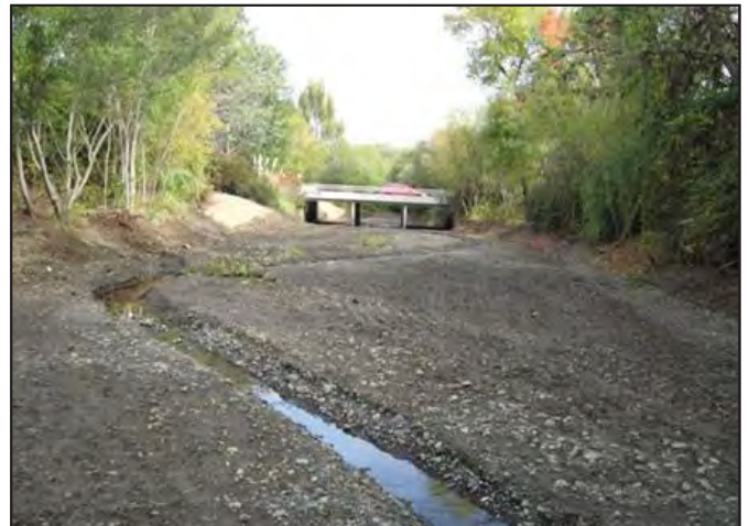
Photo d. Copeland Creek at Snyder Lane crossing, October 2008, following sediment removal activities and construction of low-flow channel.
