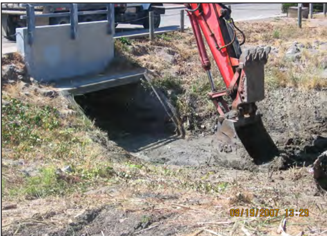
Photo e. Box culvert sediment removal staged from road crossing above.
