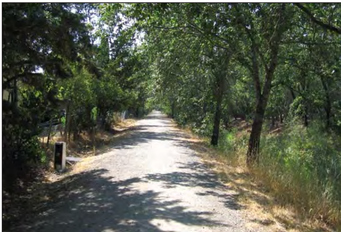
Photo a. Developed access road and v-ditch adjacent to Paulin Creek, drop inlet culvert seen in mid-ground on left.
