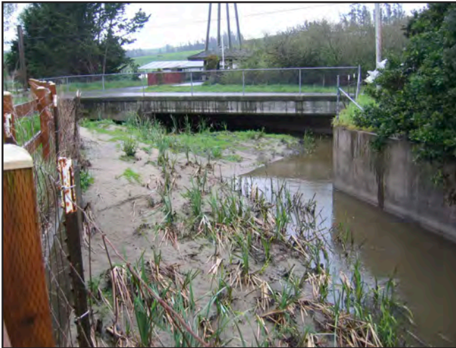
Photo a. Looking upstream at Bloomfield Channel (Zone 8A) filled with sediment.
