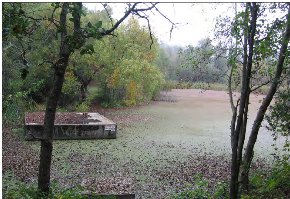
Photo b. Piner Creek Reservoir dam inlet structure surrounded by water (Zone 1A).
