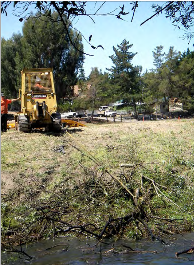
Photo c. Removing brush from creek with a sling and small tractor. Tractor remains outside of active channel.
