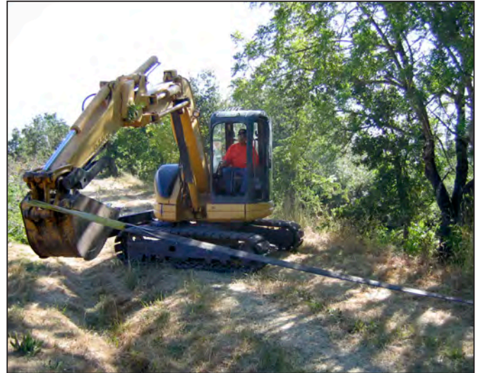
Photo b. Clearing cut brush with a sling and excavator.
