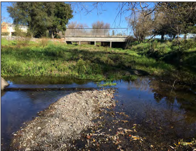
Photo c. Adobe Creek looking upstream from weir (February 2018) – chronic depositional area requiring targeted sediment removal.
