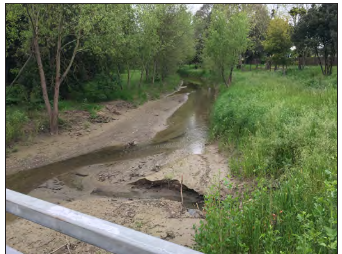
Photo d. Adobe Creek looking upstream from weir (February 2018) – chronic depositional area requiring targeted sediment removal.
