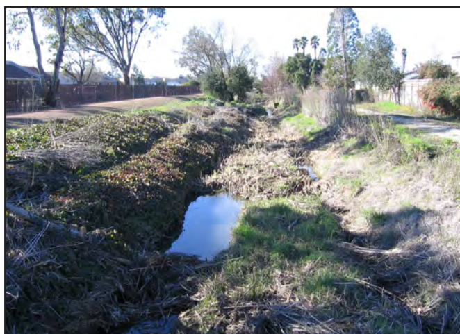
Photo d. East Washington Creek, looking downstream from Maria Drive, after cattail removal (compare to Photo c) (Zone 2A).
