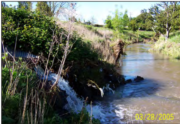
Photo a. Culvert failure on Piner Creek (Zone 1A).
