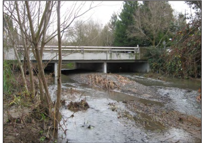
Photo b. Copeland Creek at Snyder Lane immediately following storm flows of early January 2008, 1-2 ft of sediment deposition occurs at the Snyder Lane crossing.
