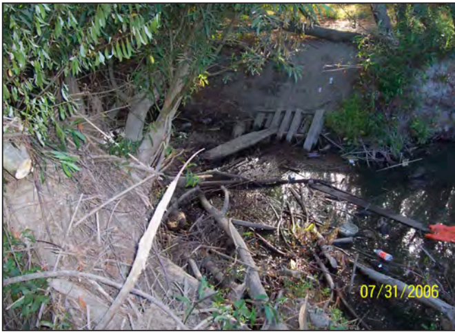
Photo a. Debris blockage in Laguna de Santa Rosa (Zone 1A).
