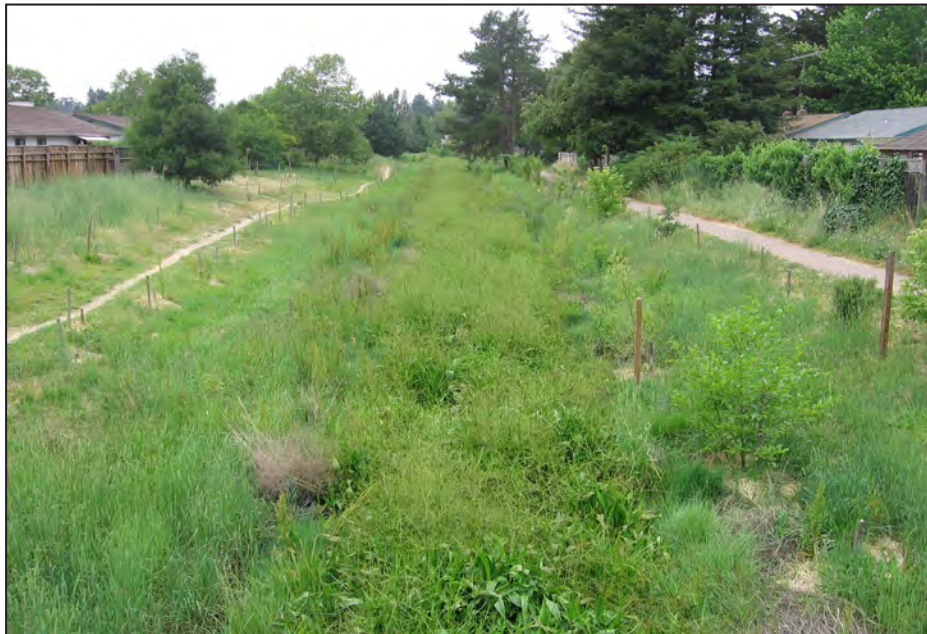
Photo b. Upper Laguna, looking downstream. Note wood stakes at top-of-bank and just up from toe-of-slope where recent planting was completed.
