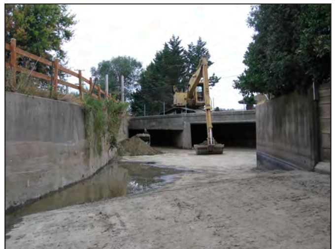
Photo d. Excavator staged on road above culvert.
