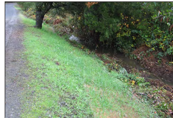
Photo b. Same site as Photos (a) after bank repair using no rock-rip rap.
