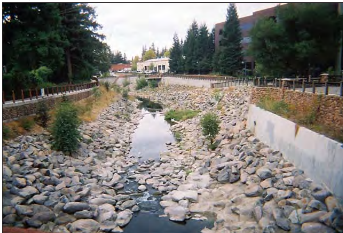
Photo b. Looking west at Santa Rosa Creek with developed pedestrian trails on both banks.
