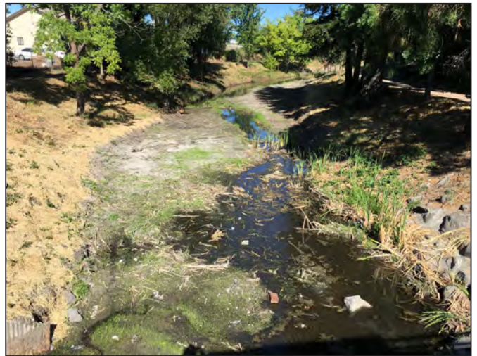
Photo d. Laguna Creek (Reach 3) looking downstream from Redwood Drive after sediment removal activities (July 2019)
