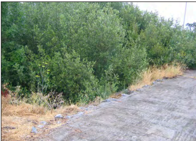
Photo e. Willows blocking culvert outlet on Windsor Creek before maintenance (Zone 1A).
