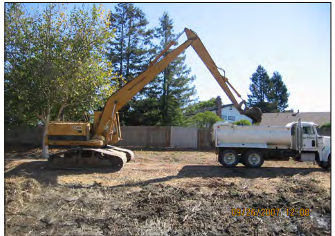
Photo d. Removed sediment placed into dump truck by excavator.
