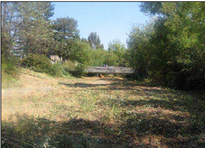
Photo c. Copeland Creek at Snyder Lane crossing, September 2008, following vegetation removal activities and prior to sediment removal activities.
